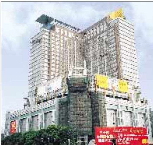
Chengdu Chuang's Centre, Chengdu, Sichuan (internal decoration works in progress)
