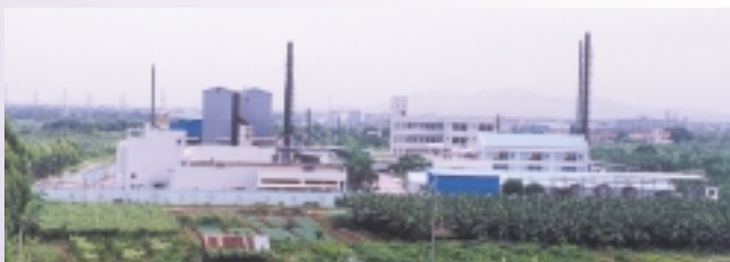
Industrial Laminate Manufacturing Plant in Zhongshan, PRC
