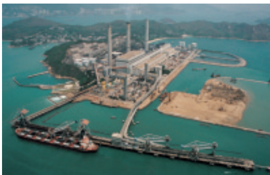
Site formation for Lamma Power Station Extension
