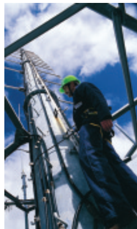
Telecommunication tower installation and maintenance
