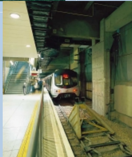
Hung Hom Station Modifications
