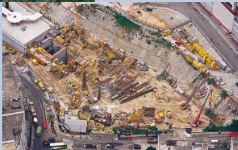
Piling Works for Tseung Kwan O Extension — Black Hill Tunnels
