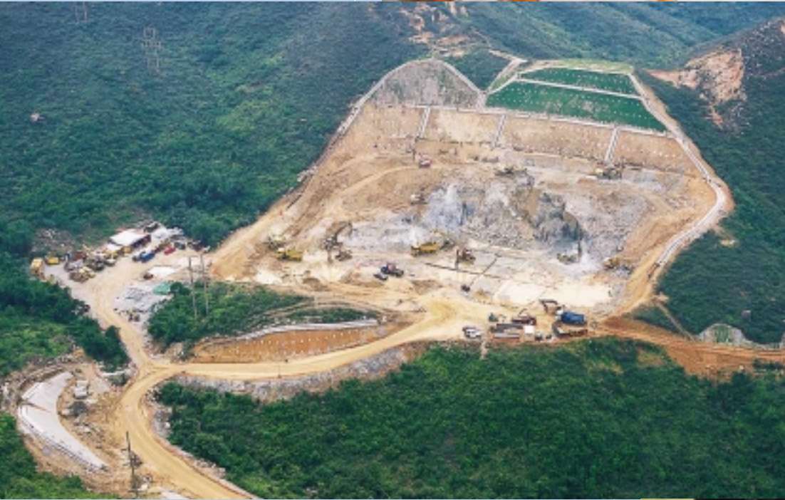
Construction of Yam O Tuk Fresh Water Service Reservoir
