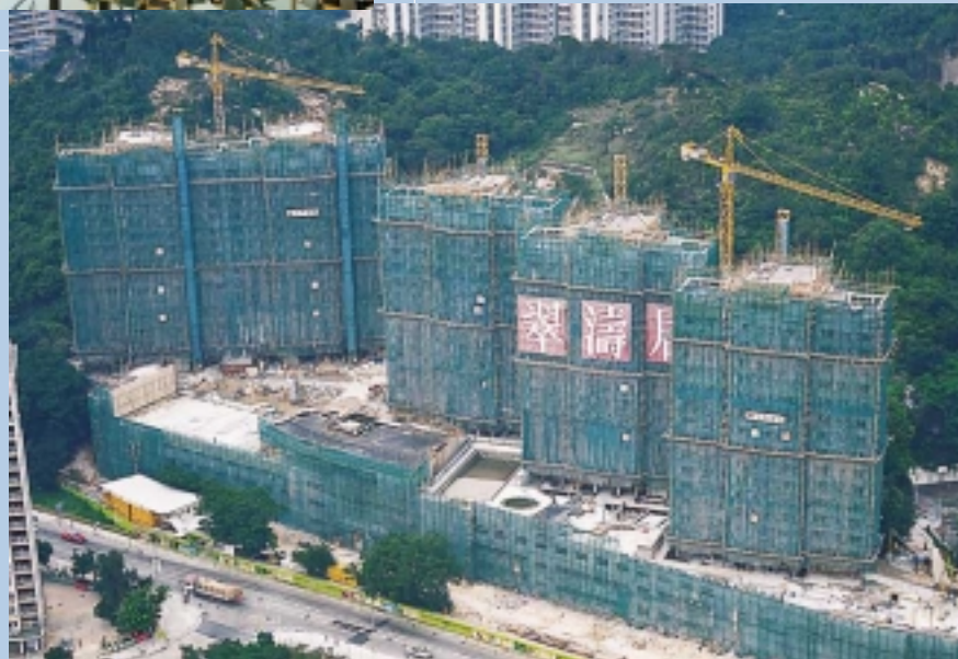
Residential Development at TMTL 386, Tuen Mun
