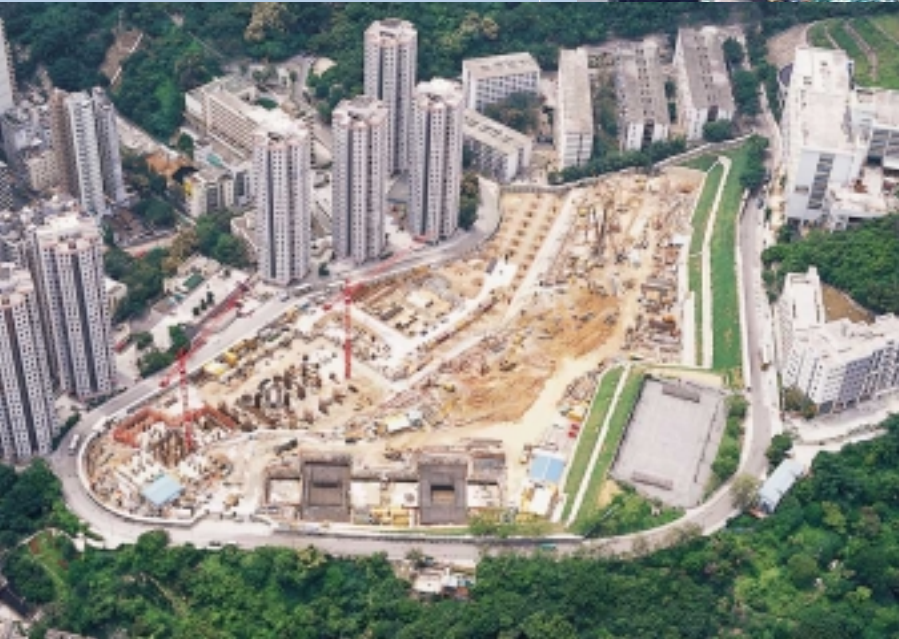
Foundation for Redevelopment of Shek Pai Wan Estate Phase 1
