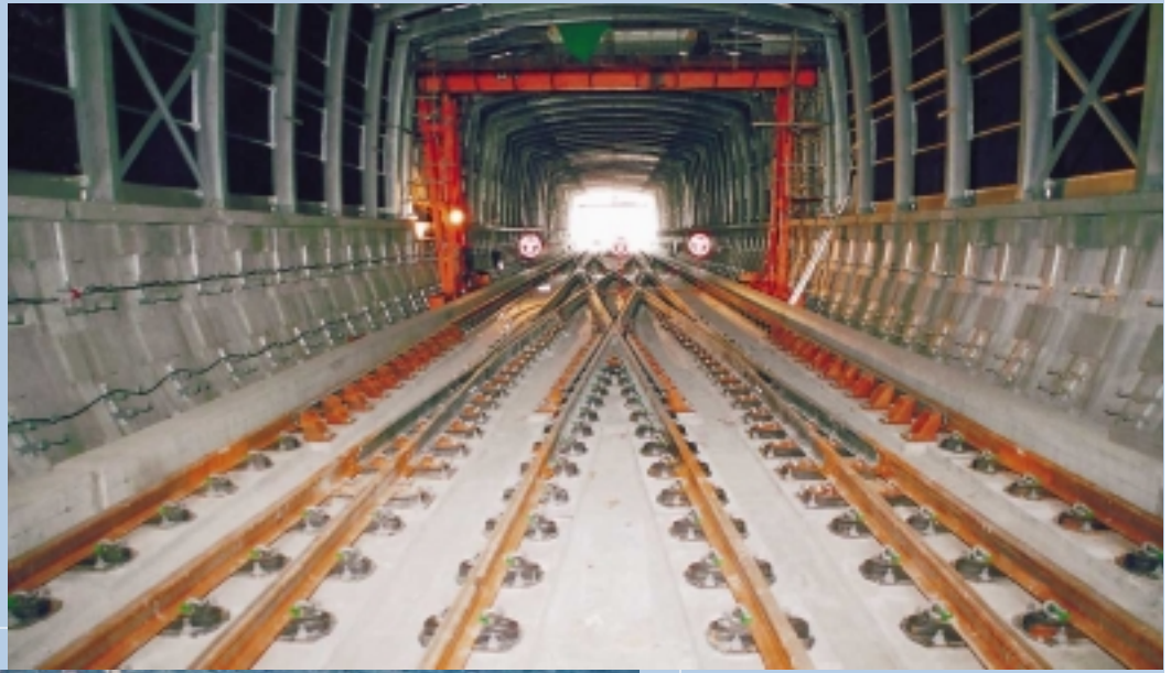
West Rail Permanent Way — Northern Area
