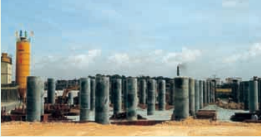
Construction of the Guangzhou-Zhuhai West Superhighway (Phase I)
