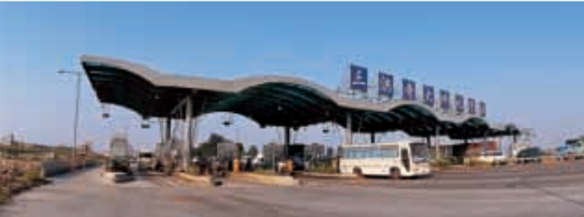
Toll station at Sanhongqi Bridge
