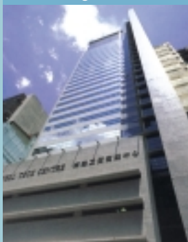
Well Tech Centre, San Po Kong
