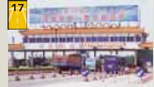
Roadway No. 321 (Deqing Section)
