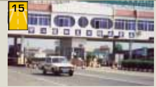
Roadway No. 1964 (Zhaojiang Section)
