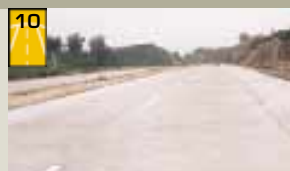
Roadway No. 1906 (Qingcheng Section)
