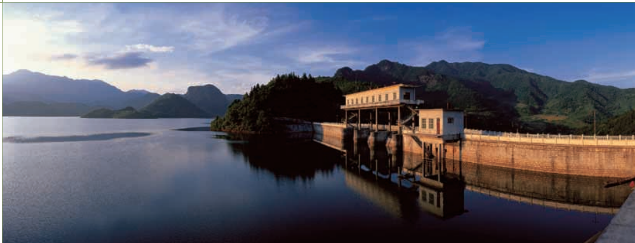
Xiaozhu power station, part of the Huaiji Power Project
