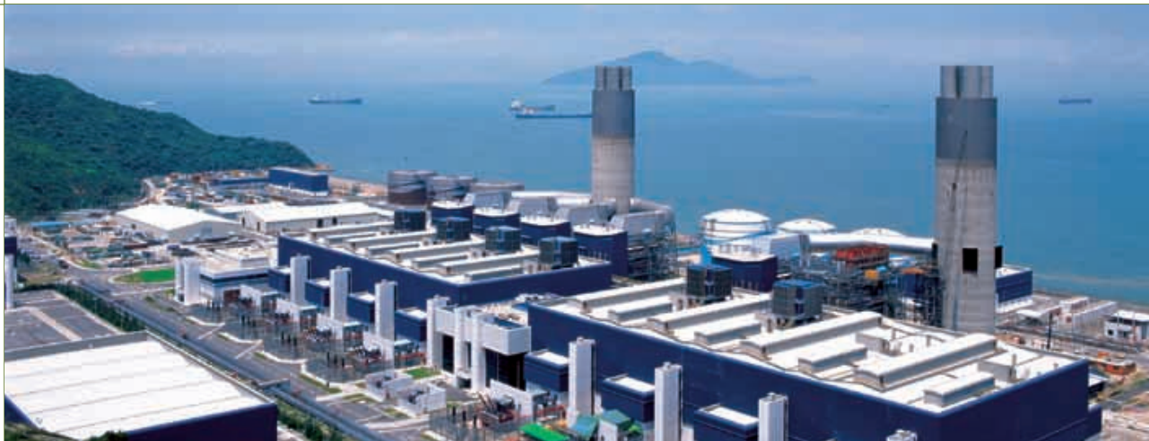
Black Point Power Station
