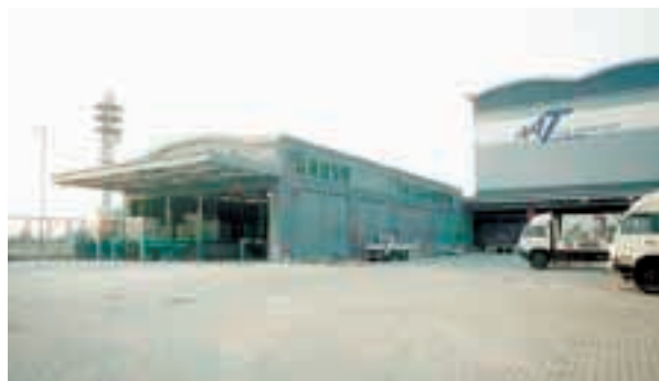
Western-By-Pass facility at Asia Airfreight Terminal
