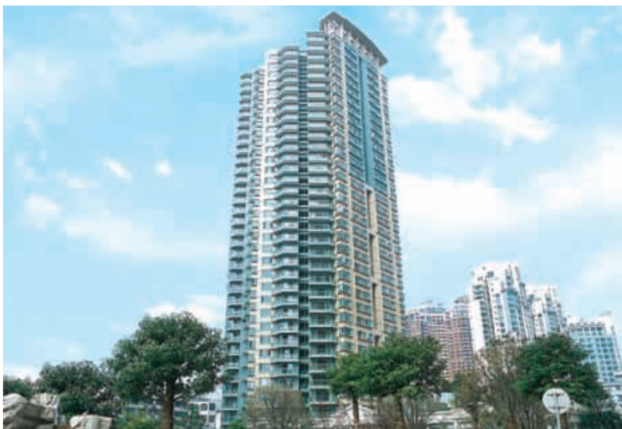
Central Residences Tower 5, Shanghai, PRC
