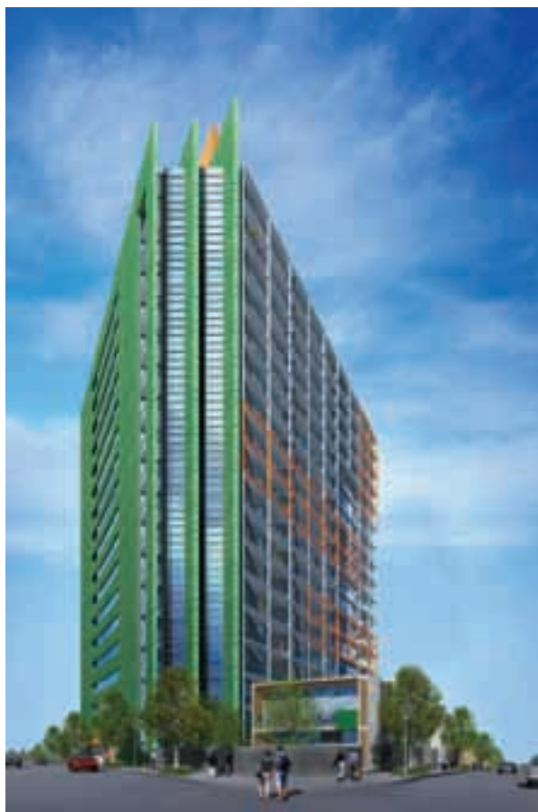
The Quarry at Jacksons Landing, Sydney, Australia
