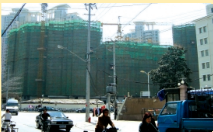
Phase II of Fragrant Garden in Shanghai is under construction
