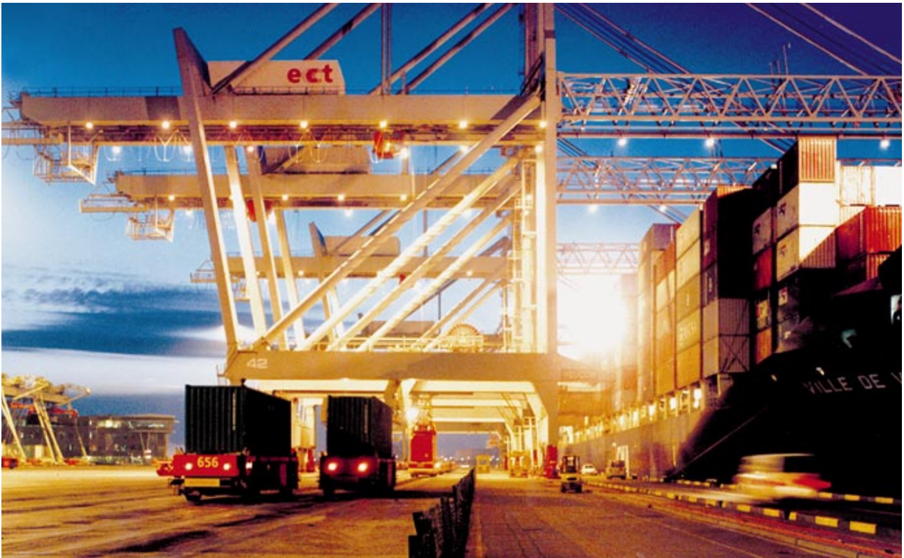
A view of the automated ECT Delta Terminal at nightfall where the automated guided vehicles are discharging a vessel.
