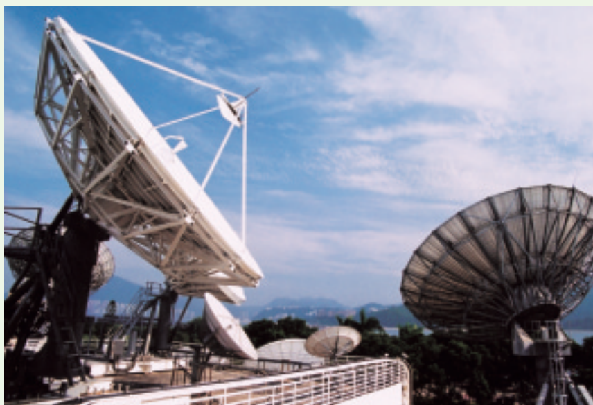
The newly installed satellite TV broadcasting facilities in the Satellite Control Centre Phase II has started to provide satellite TV uplink and broadcasting services via its satellite TV broadcasting platform. It can operate up to 18 satellite TV channels.
