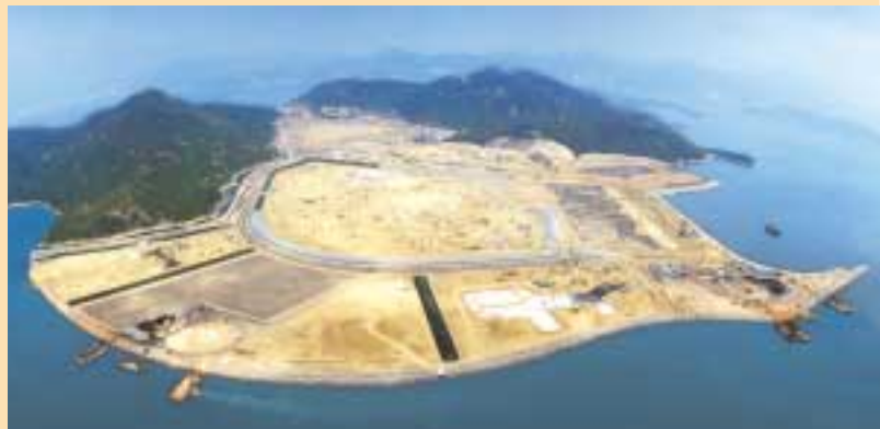
Phase II Infrastructure of Disneyland at Penny's Bay
