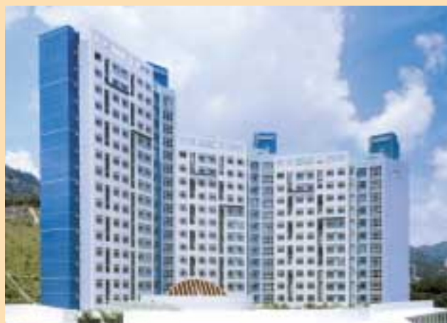
Student Hostel Phase 1, NKIL 6284 Cornwall Street, Kowloon
