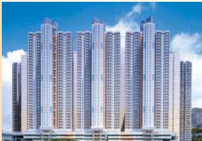
HOS at Po Lam Road Housing Development Phase 3
