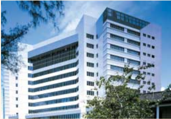
Kowloon Hospital Phase 1 Redevelopment at Mong Kok, Kowloon
