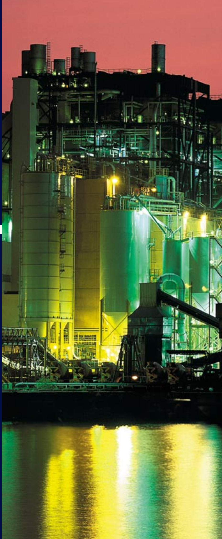
Lamma Power Station at night showing important environmental protection facilities: ash silos (foreground) and boilers fitted with low NOx burners (background).
