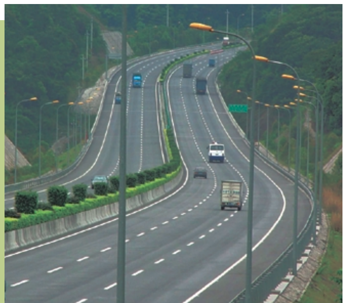
The recently completed Guangzhou Northern Second Ring Expressway
