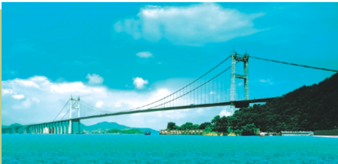
Humen Bridge connecting the eastern and the western sides of the Pearl River Delta
