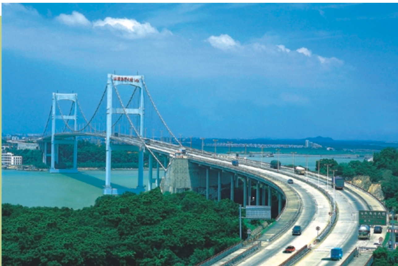
Shantou Bay Bridge acquired in July 2002
