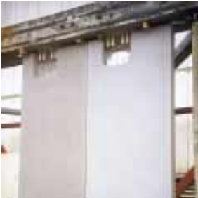
Conduits embedded into panel
