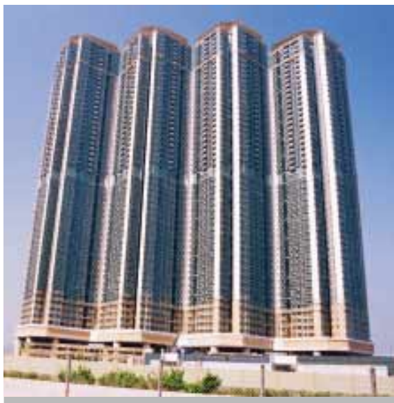
Caribbean Coast, Tung Chung Over 30,000m 2 of YTONG Panel are being used as internal partition wall to replace conventional concrete block wall
