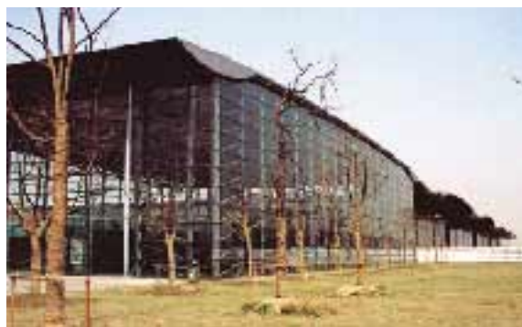
East Elevation of Entry Hall and Exhibit Halls 入口廳和展廳的東側面
