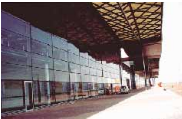
Steel Structures for Exhibit Halls 展廳鋼結構
