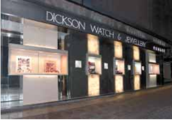
The newly-renovated Dickson Watch & Jewellery shop at The Landmark. 位於置地廣場經裝修後的「迪生鐘錶珠寶」精品店。
