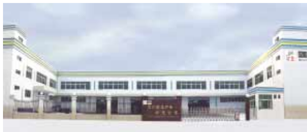
Yuanzhou plant extension
