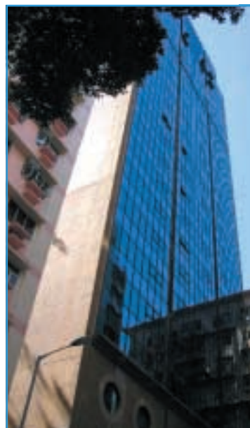
Hon Kwok TST Centre at 5-9 Observatory Court, Tsim Sha Tsui, Kowloon
