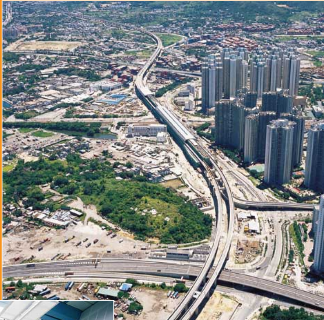
West Rail Phase 1 – Construction of viaducts
