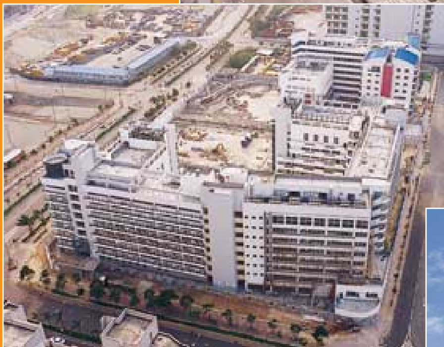
Construction of three schools at Fat Tseung Street, Sham Shui Po
