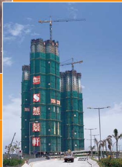
Vianni Cove at Tin Shui Wai Town Lot 27, Yuen Long
