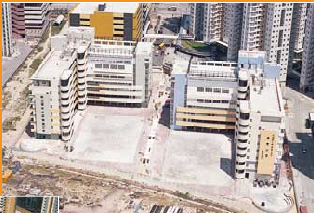
Construction of two primary schools at Tin Shui Wai Area 111
