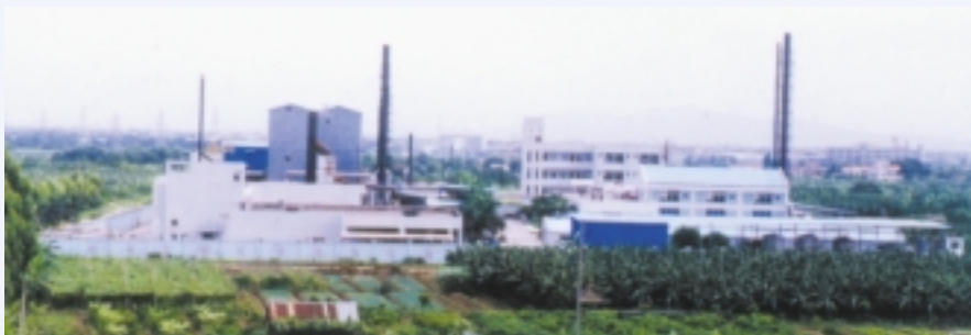
Industrial Laminate Plant in Zhongshan, the PRC
