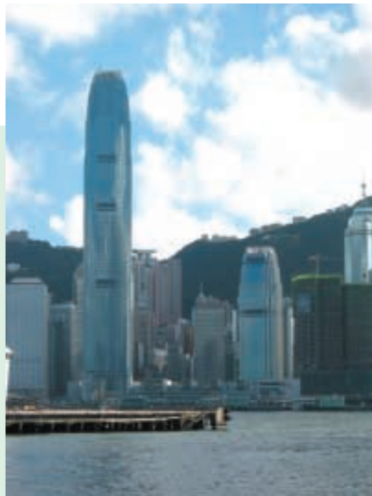
Supply and Installation of ELV Systems includes Digital CCTV Surveillance Systems, Security System, Giga-bit Ethernet fibre backbone, SMATV, Walkie Talkie, Radio Paging System and Public Address System at Two International Finance Center, the 88-storey class A intelligent commercial building at Central
