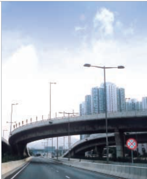
Tin Shui Wai Further Development (Tin Ying Road and Tin Tsz Road External Links)
