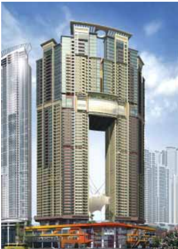
Airport Railway Kowloon Station Package 3 will have over a million square feet of luxury residences.
