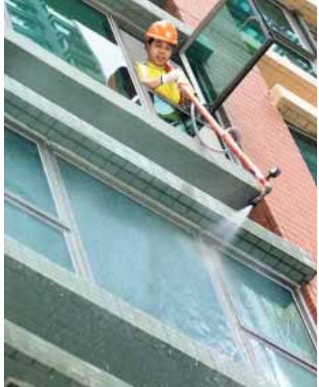
The Group tests every window in new developments with a high-pressure water spray after installation.
