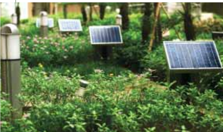
The Parcville in Yuen Long is Hong Kong's first environmentally-friendly estate and a showcase green project. Shown: Solar power illuminates the landscaped garden.
