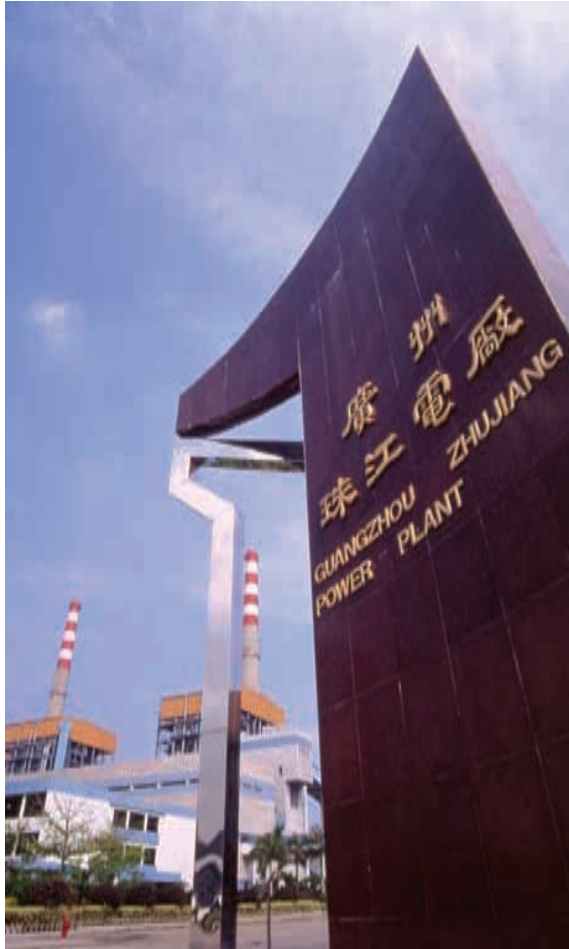
Zhujiang Power Station has the largest power generation capacity in our Energy Division.
