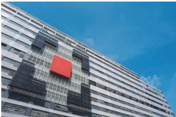
ATL Logistics Centre is the world's first and largest intelligent multi-storey drive-in cargo logistics centre.
