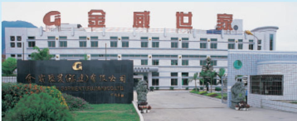
Exterior of the Group's production facilities at Putian City, Fujian Province
