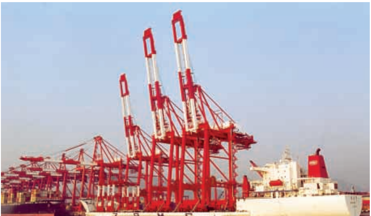
New berth of Chiwan Container Terminal, Shenzhen, PRC
