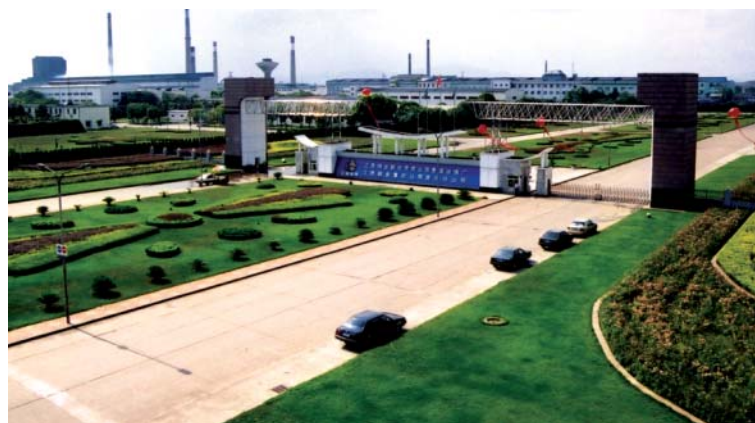
Guixi Smelter — the largest smelter with state-of-the-art technology in the PRC
