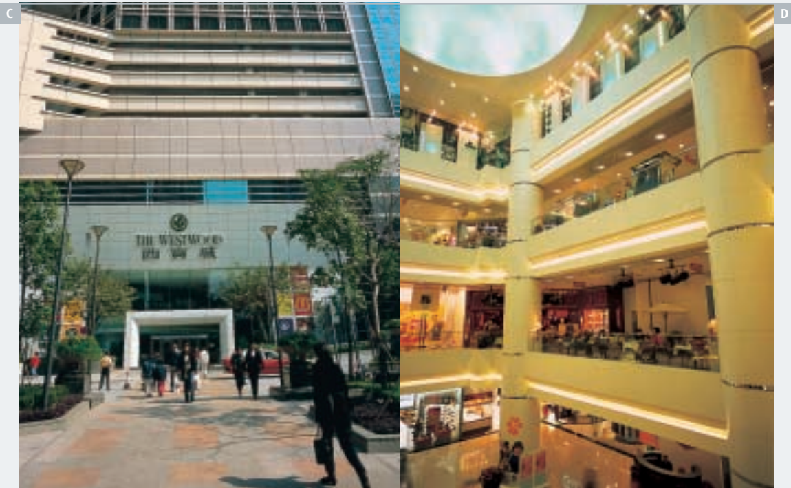
Shanghai Liu Chong Hing Financial Centre A. Prospective view B. Construction site status The Belchers’ C. Entrance of shopping arcade D. Inner view of shopping arcade
