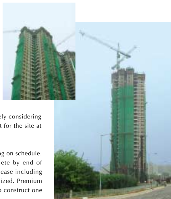
Fanling Sheung Shui Town Lot No. 189 55% owned by the Group, the construction work of this site is underway for three 40-storey residential towers. Total gross floor area of the development will achieve approximately 45,120 sq.m. with 139 carparking spaces.
