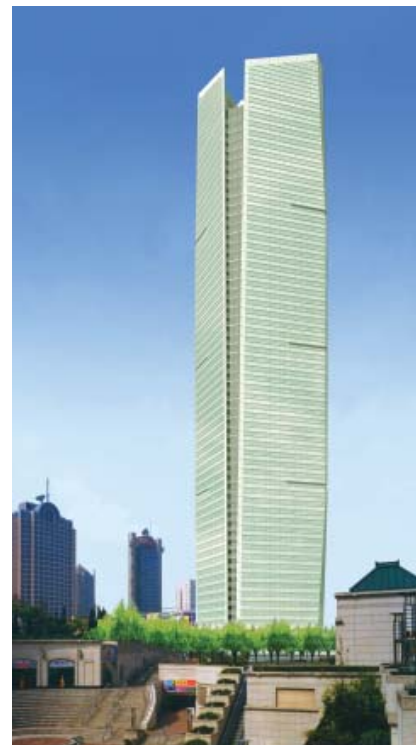
Shanghai Wheelock Square, one of the Group's commercial property developments, is slated for completion in 2007.
