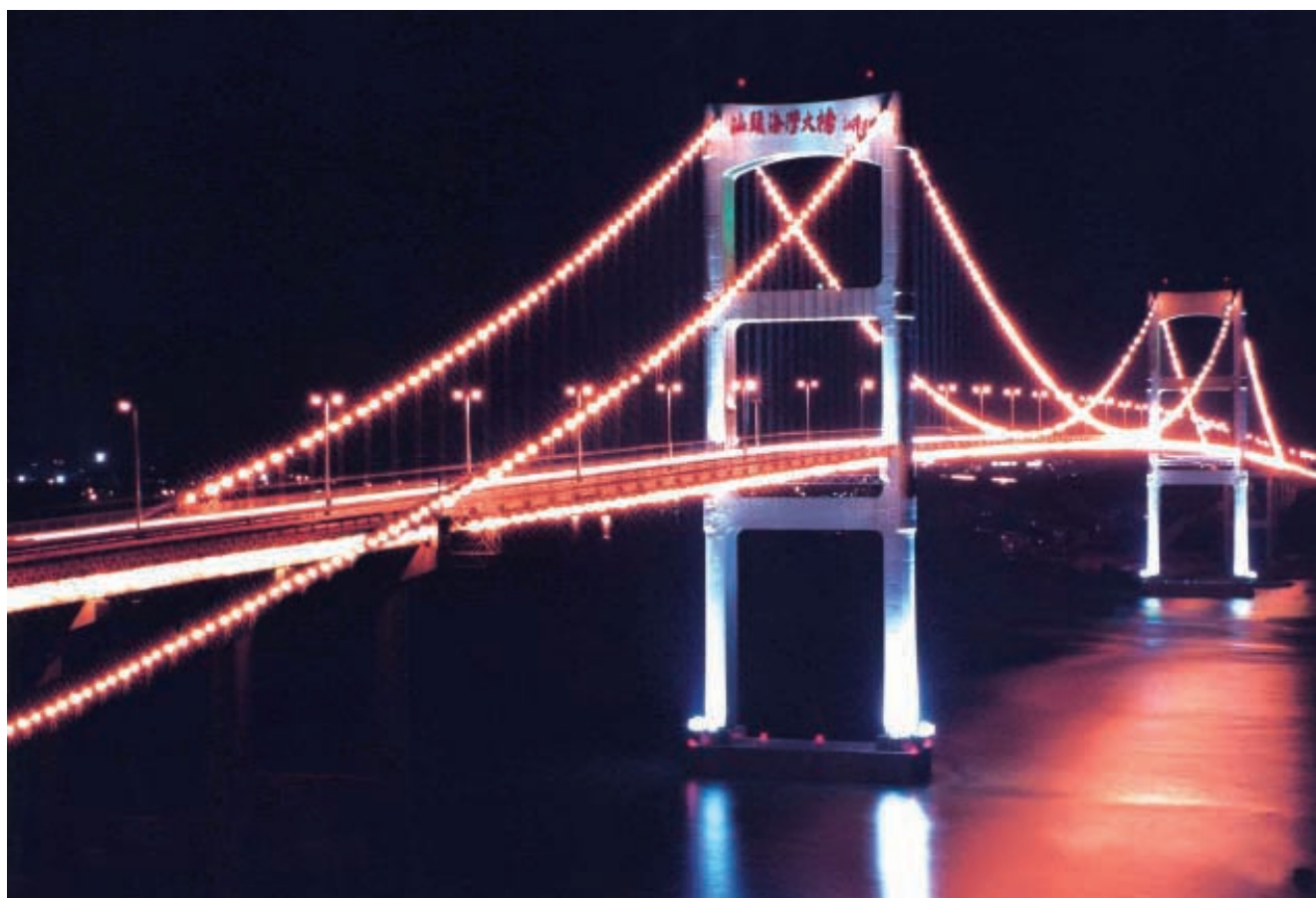
Shantou Bay Bridge
