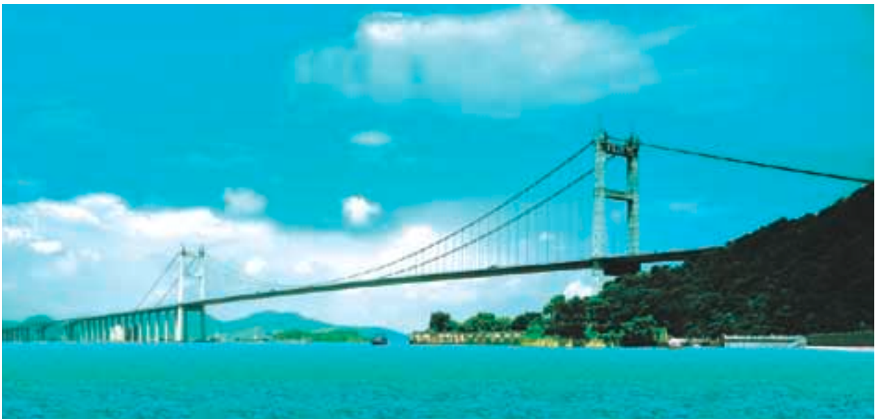
Humen Bridge connecting the eastern and the western side of the Pearl River Delta
