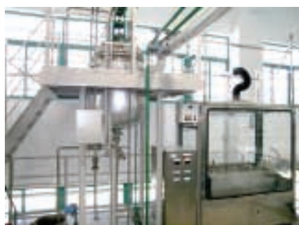
The Chemical Plant in Zhuhai
