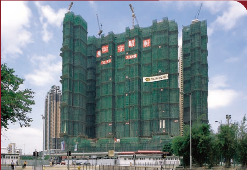
The Pacifica at NKIL 6275 West Kowloon Reclamation
