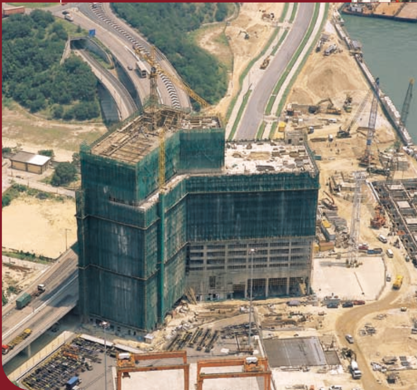
Office Building at TYTL 139, Tsing Yi
