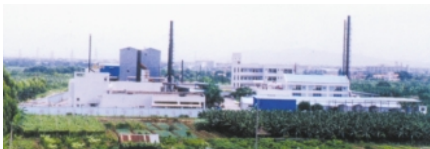
Industrial Laminate Plant in Zhongshan, the PRC
