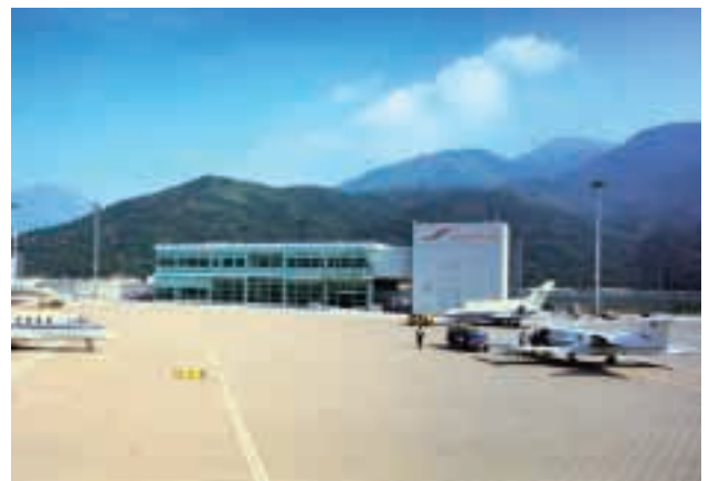
The Hong Kong Business Aviation Centre is Asia's premier executive aviation support facility.
