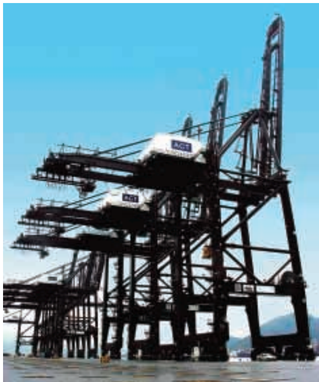
Asia Container Terminals has swapped the two berths at Terminal 9 for two existing ones at Container Terminal 8.
