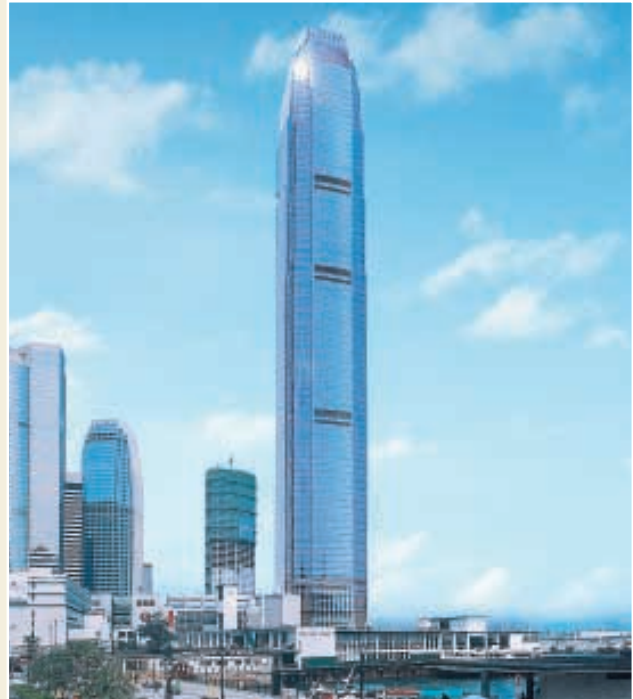
International Finance Centre, Central, Hong Kong
