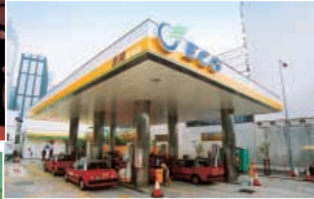
ECO-Liquefied Petroleum Gas Filling Station
