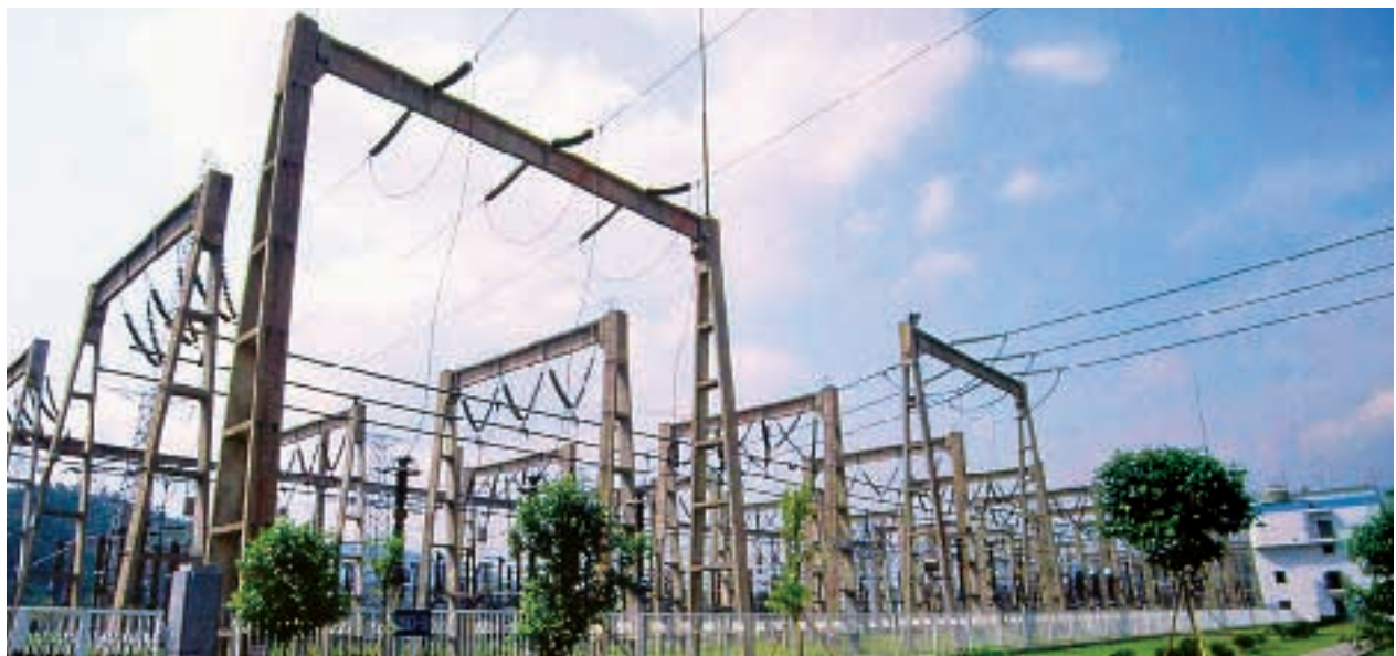
Zhujiang Power Station
