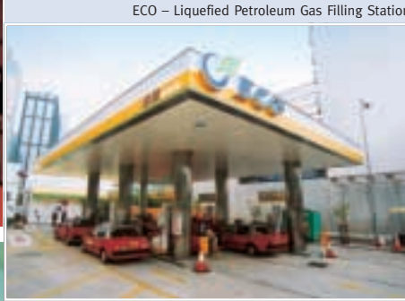
ECO – Liquefied Petroleum Gas Filling Station
