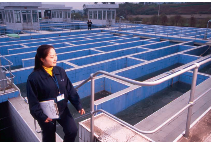
Chongqing Water Plant supplies water to thousands of homes and businesses.
