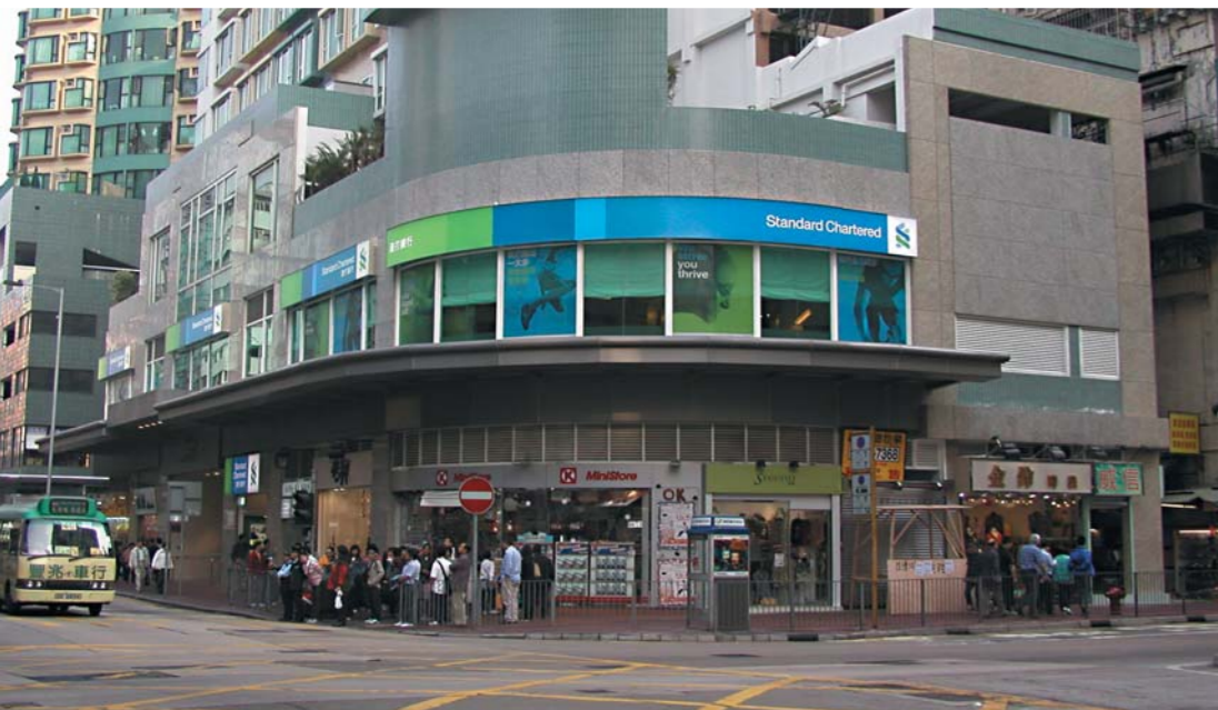
Shops at Bijou Apartments, Mongkok 旺角別樹華軒之商舖
