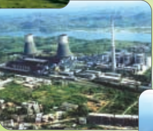
Guixi Power Plant
