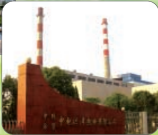
Hongze Power Plant
