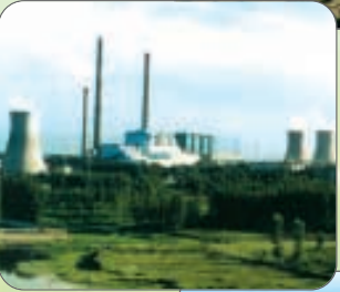
Shentou I Power Plant
