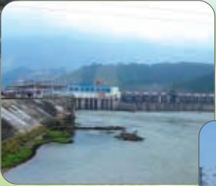
Shaxikou Power Plant
