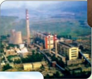
Qinghe Power Plant
