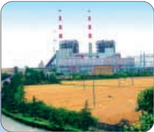
Pingwei Power Plant
