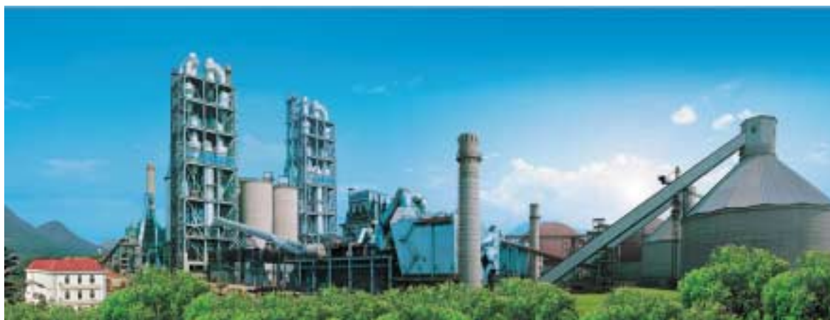
The two clinker production lines with a daily production capacity of 10,000 tonnes located in Tongling, Anhui
