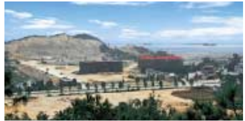
Jiangmen Conch under construction
