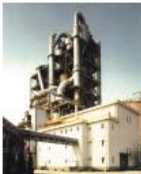
Waste-heat electricity generator
